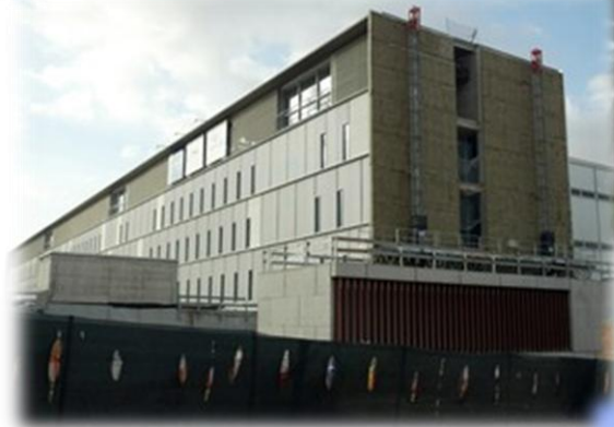
Hospital Baix Lobregat
