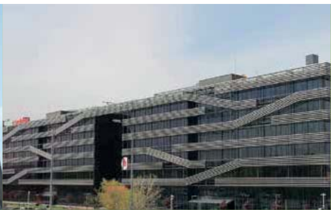
VODAFONE MADRID 2013/2014 Cooling Capacity KW 1.032 Close Control N° 68 Units ED.X
