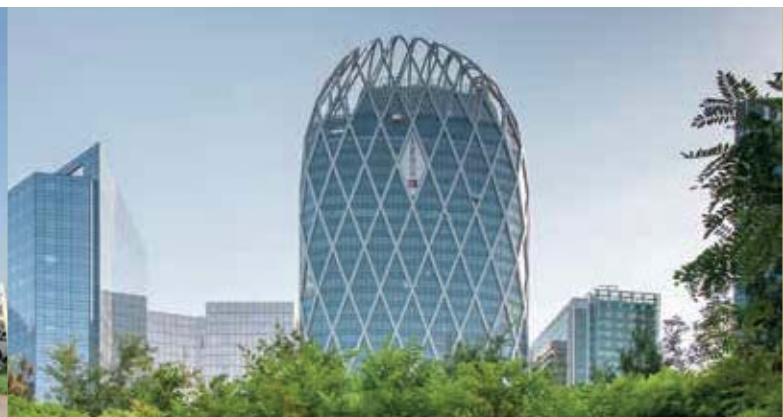
TOUR D2 PARIS 2012 Cooling Capacity KW 475 Close Control Unit N° 8 Units UW
