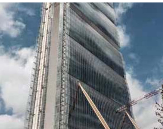
ISOZAKI MILAN TOWER 2014/2016 Cooling Capacity KW 1.310 Close Control Unit Model N°7 Units ED.X + N°49 Units EDH
